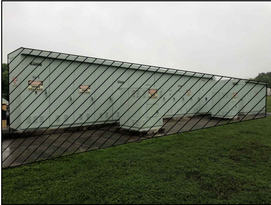
Exist. Switchgear and Vault Demolition
