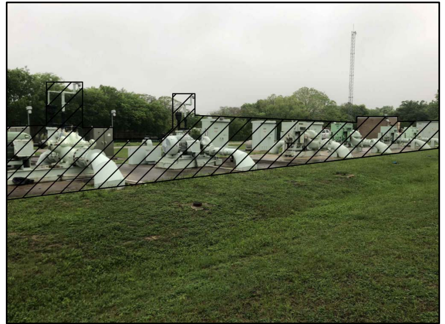
Exist. Pump Station Pumps and Pad Demolition
