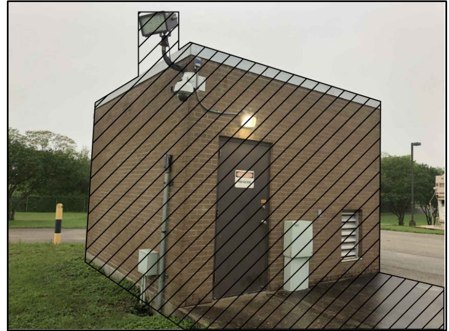
Exist. Electrical Building Demolition
