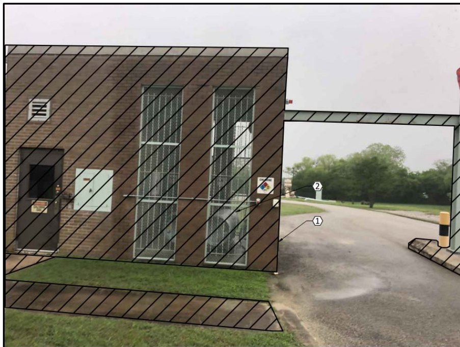
Exist. Chlorine System Facilities Demolition
