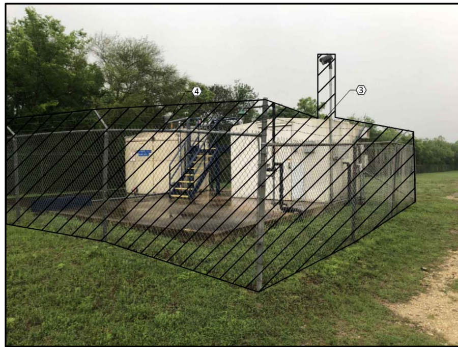
Exist. Fluoride System Facilities Demolition
